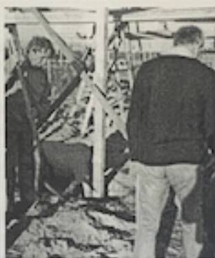
DIGGING THE FOUNDATIONS, GERRY SPENCER SUPERVISES RON TODD
