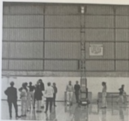
ROTARIANS COMMENCE THE TRANSFORMATION OF BASKETBALL COURTS AT SURFSIDE CENTRE
