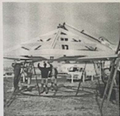
ROOF FRAME OF ROTUNDA LIFTED INTO POSITION BY MOBILE CRANE
